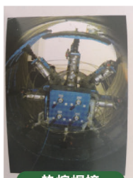
热熔焊接 Hot Melting Tape Connection
